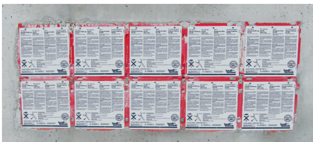
double wall insert HSI 150 as block used in formwork
