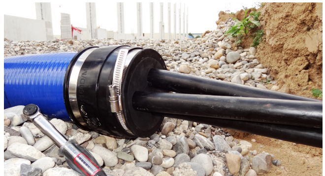
sealing in soil at the end of spiral hose Hateflex 14150 with the sealing set KES-M 150 WE 160-SG-3/22-54
