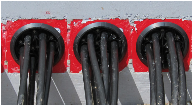
low-voltage cables sealed with HSI 150-DG-6/10-36
