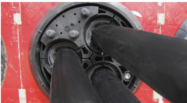
pressure plate cover HSI 150-PA-3/24-54
