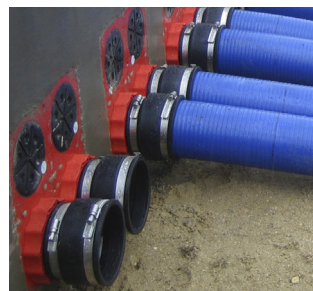
pressure-tight connection to HSI 150 wall inserts
