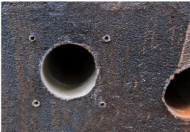
core drill and dowel holes
