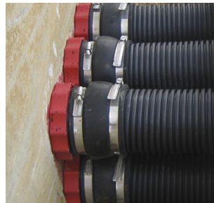
connection of corrugated pipes with sleeve method HSI 150-M 168
