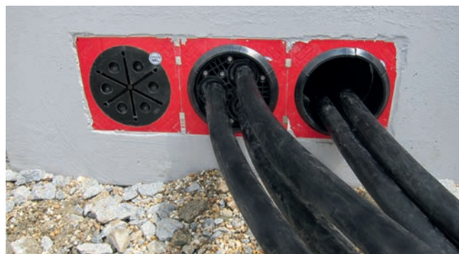
various installation stages for HSI 150-DG-3/24-54
