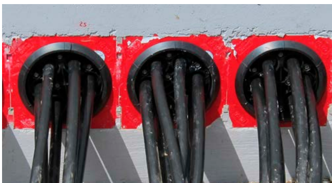
low-voltage cables sealed with HSI 150-DG-6/10-36
