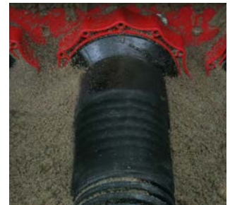
connection of corrugated pipes with cold shrink sleeves HSI 150-D 110-KS
