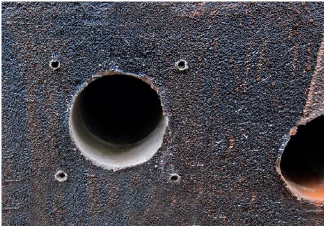
core drill and dowel holes
