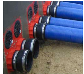
pressure-tight connection to HSI 150 wall inserts
