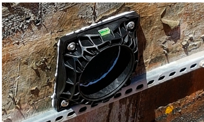
HSI 150-DFK Wall flange and sealant was placed over the core-hole and is fixed using watertight screws and dowels.
