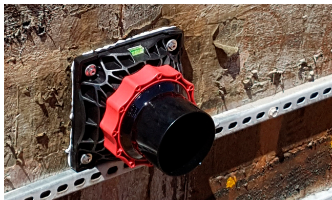
HSI system cover is then simply attached via the bayonet system to the DFK and tightened by the red clamping nut.
