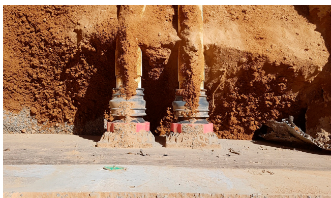
Conduit is then connected using the rubber connection sleeve that comes with the system cover.
