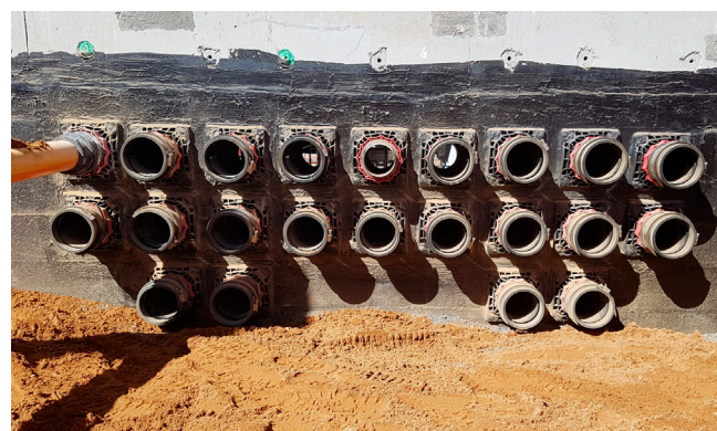
KME trialled three to begin with, the builder then approved the system and completed another layer of the membrane. New core-holes were drilled then another twenty two HSI 150-DFK and system covers were installed after early success and ease of installation.
