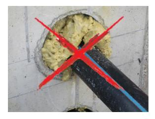
Ad-lib sealing solutions of the can are often not showing the desired result and hold a serious
