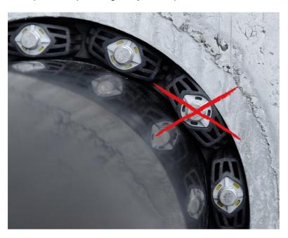
As the nuts are moulded into the bottom pressure plates they cannot get lost during installation.
