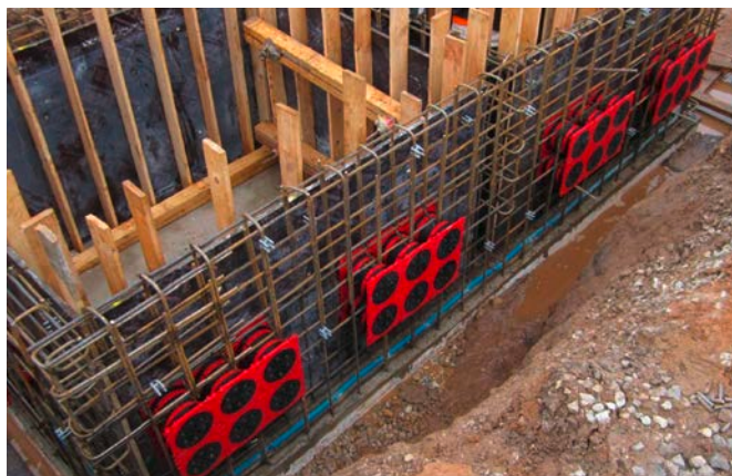
several packages HSI 150-K2 in manhole
