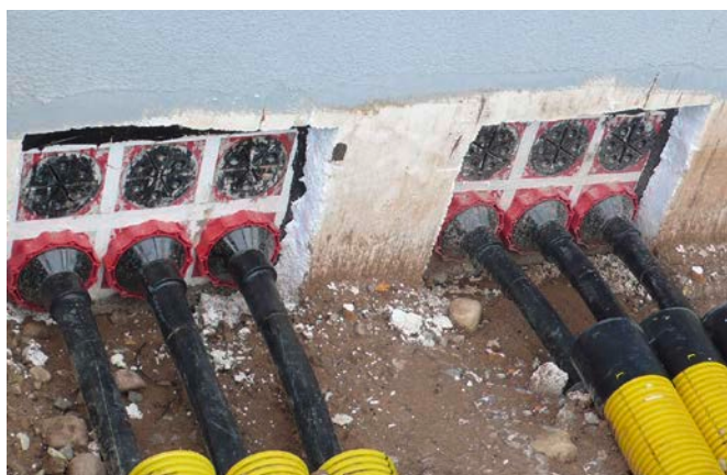
cable sealing with heat shrink method
