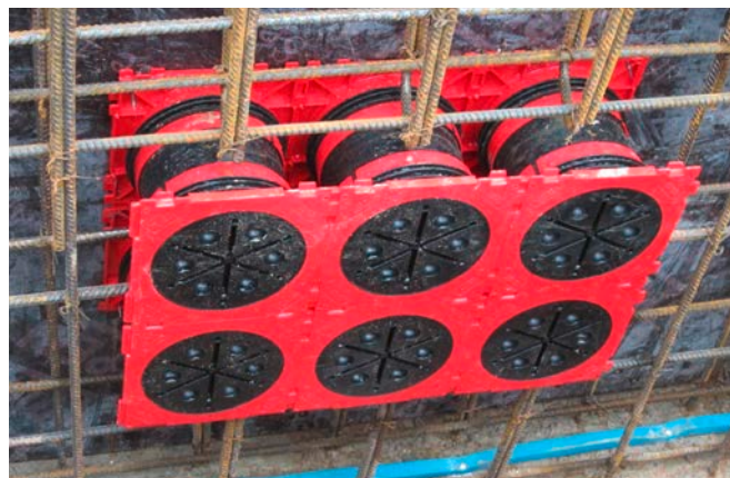
double wall insert HSI 150-K2 fixed as a package into the formwork
