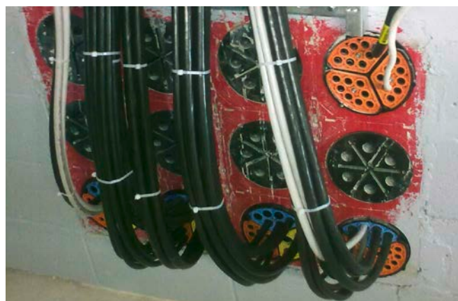
cable sealing with SEGMENTO
