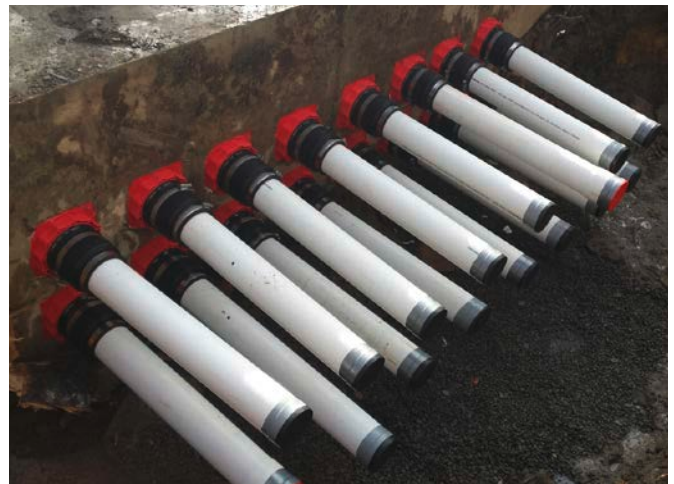
connection of rigid Telstra conduits to HSI 150 wall inserts using KES-M 150-D system cover
