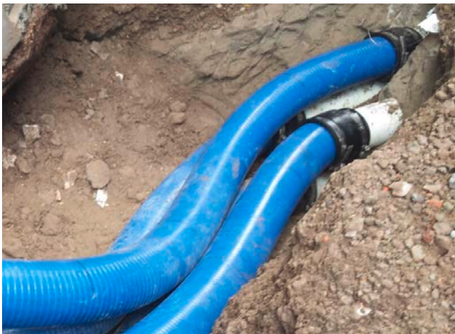
connection of Hateflex spiral hose to rigid Telstra conduits
