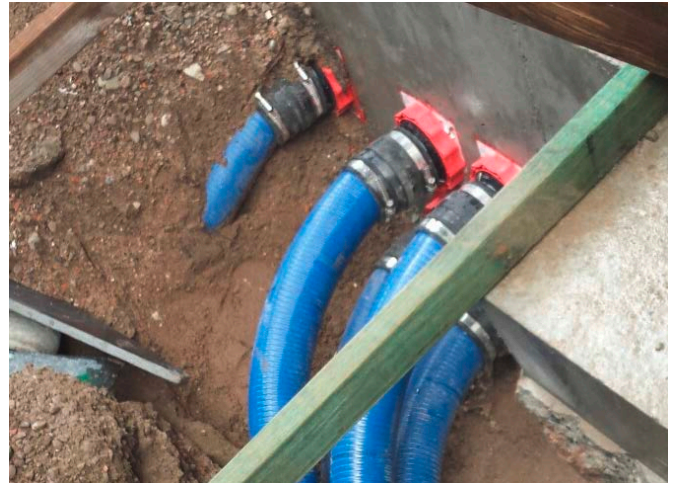
connection of Hateflex spiral hose using KES-M 150-D system cover
