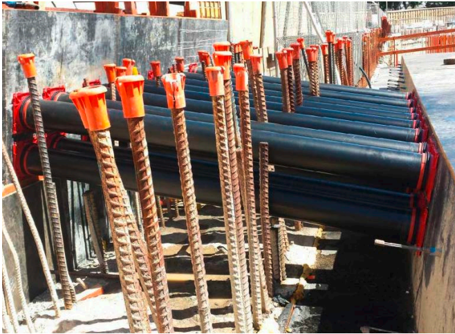
HSI 150-K2 wall insert 2,100 mm – mounted in formwork
