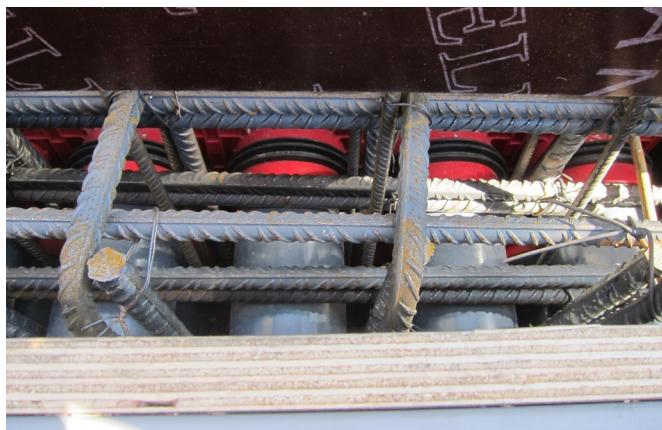
HSI 90 before pouring the concrete
