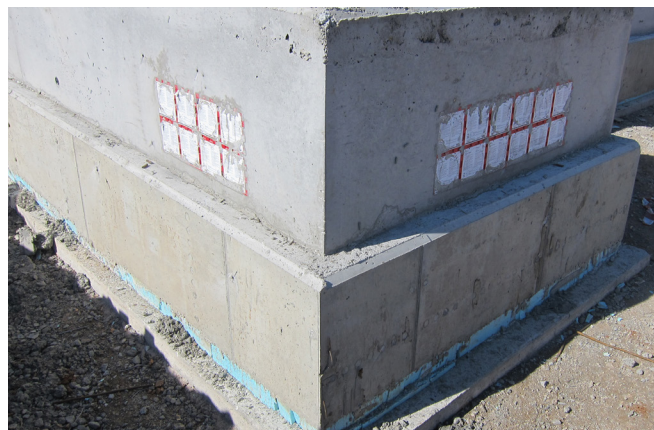
HSI 90 after removing the formwork
