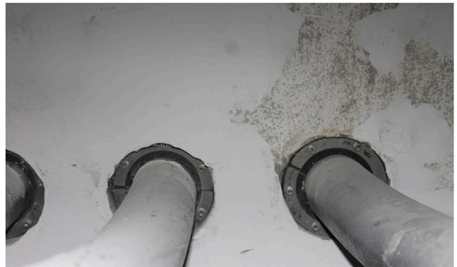
As a unique solution, Hauff-Technik cable mechanical seals with their numerous advantages are used. The core holes are now water-resistant and therefore perfectly suitable for the location area. Additionally, the mechanical seals with the segmented ring technology allows individual cable diameters to be fit in as well as ensuring the central alignment of the cables. In summary, the client received a professional and a clear solution to the individual requirements.
