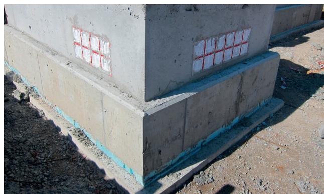
HSI 90 after removing the formwork
